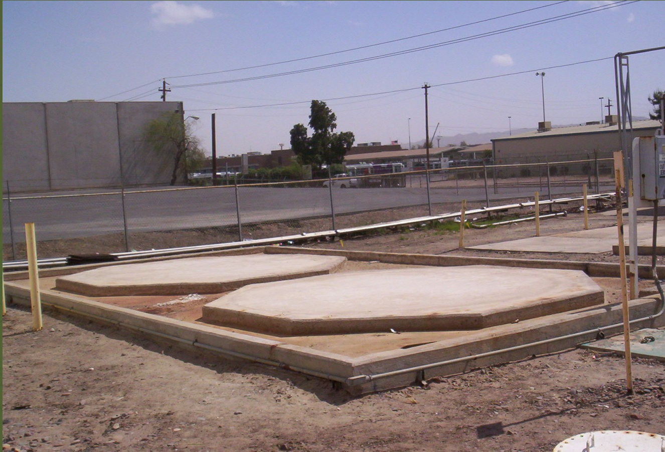
Foundation for new tanks
